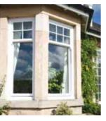
Complete with runthrough horns that recreate the look of a traditional box sash. with a mechanical joint option, our vertical sliding sash windows are the perfect replica, with the added appeal of being maintenance-free and energy efficient.
